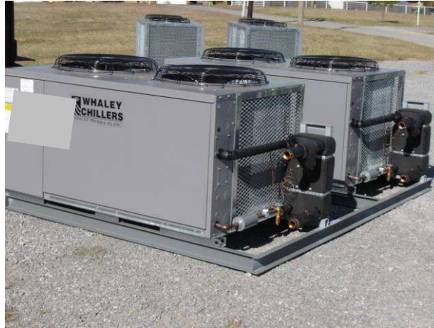
Figure 32. Compressor chiller ( http://www.liquidchillers.org )
