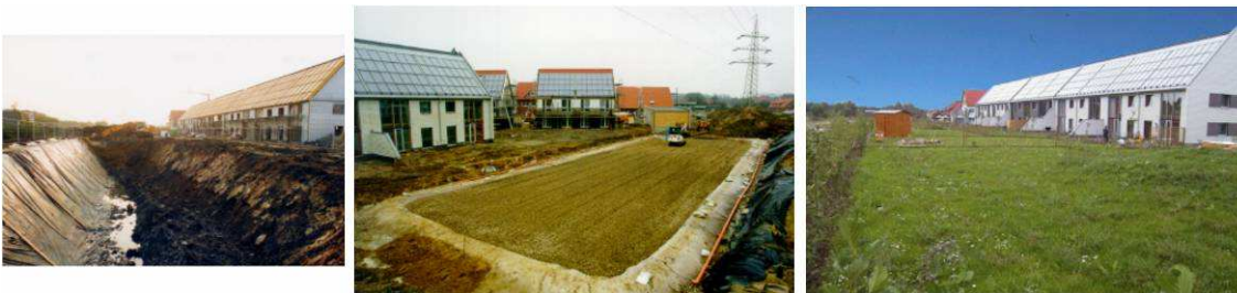
Figure 62: Example of a GWTES realization in Steinfurt, DE, with from left to right: excavation of the storage volume, filling of the storage pit with gravel and heat exchanger mesh and fully covered thermal energy storage [24].
