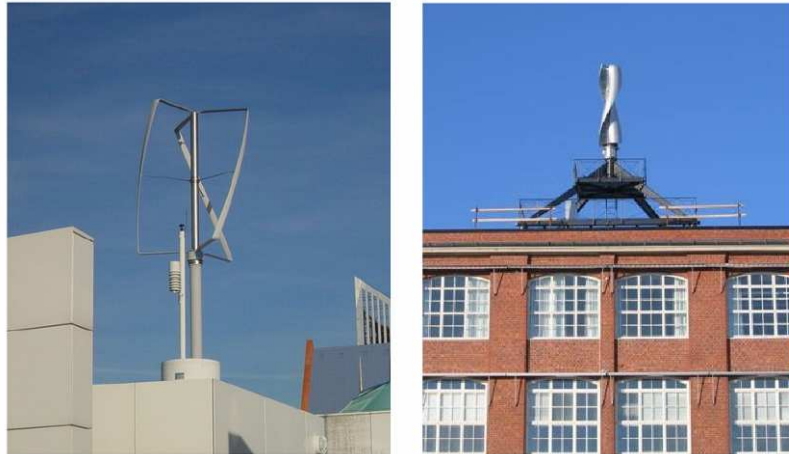
Figure 10. Vertical axis wind turbines
