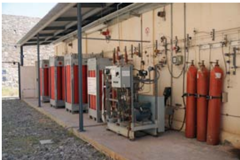
Hydrogen storage and distribution grid.
