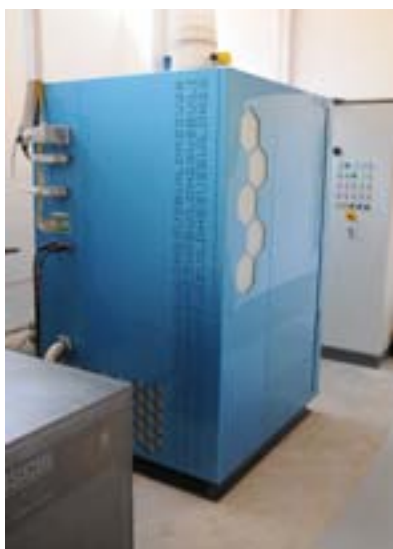
Fuel cells based 20kW micro-cogeneration system
